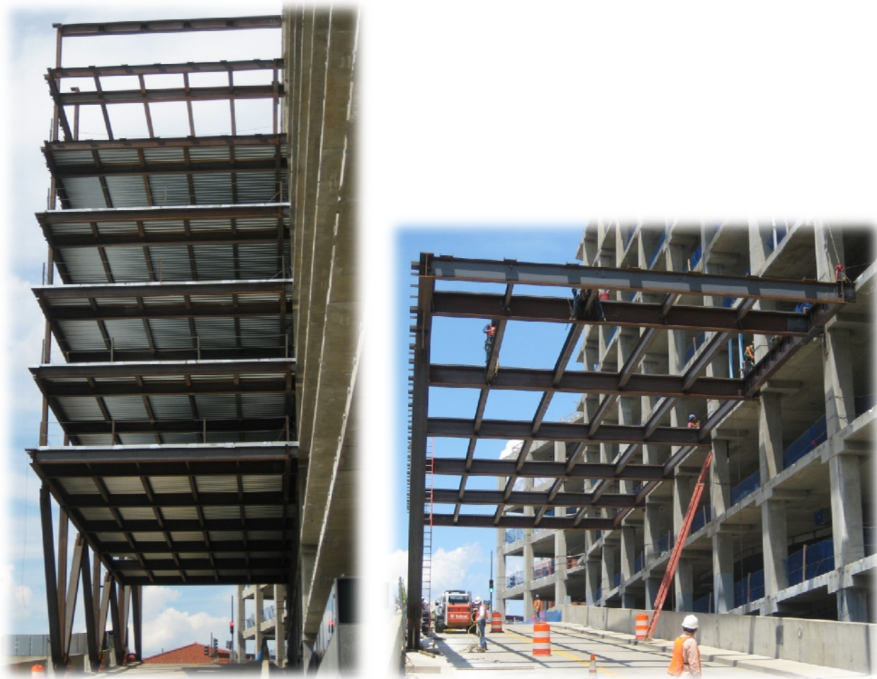
Figure 4 & 5: the M Street Ramp Steel Structure
